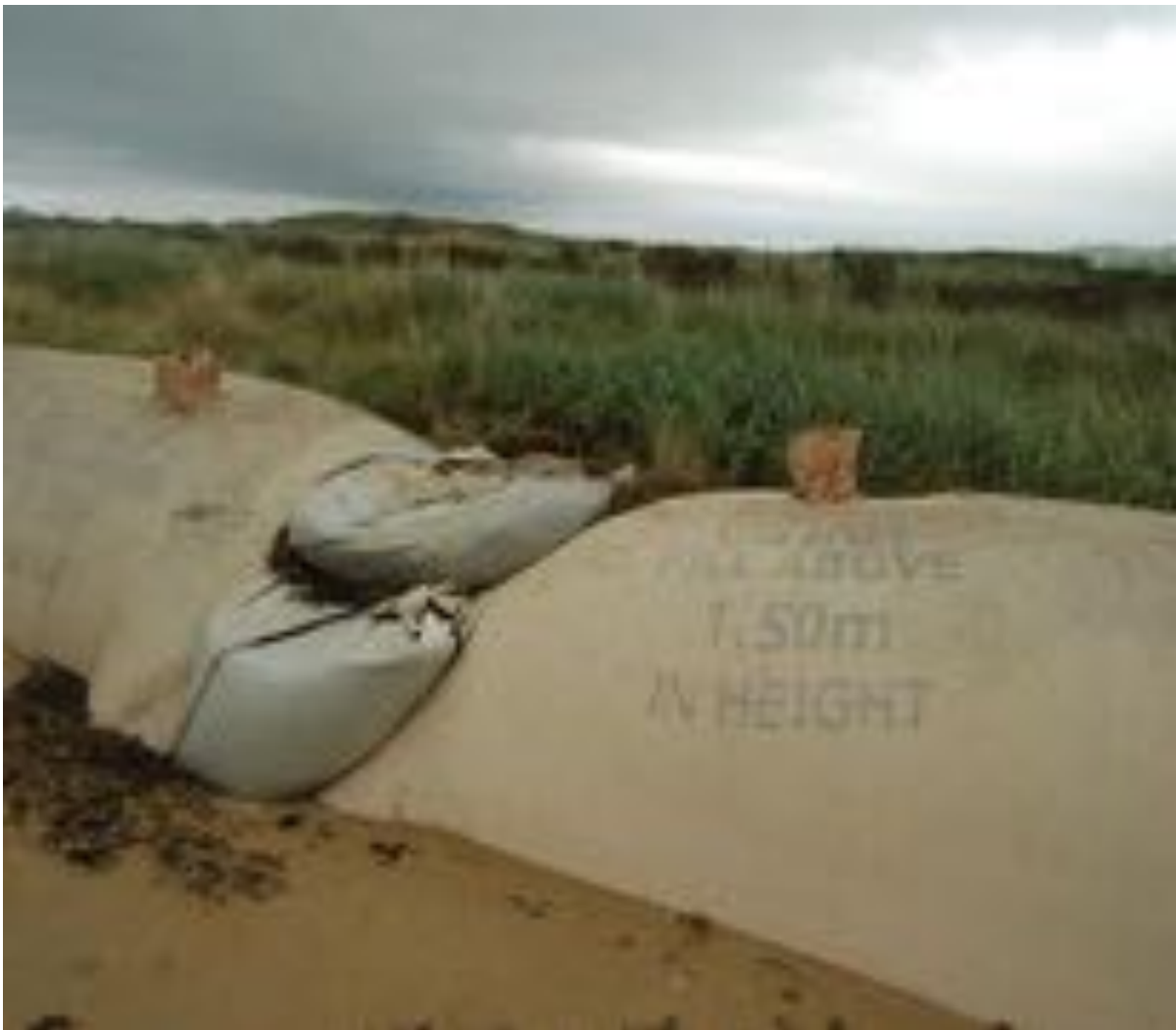
Sand-filled geotube, Donegal Boardwalk Resort, Carrickart, Donegal — Republic of Ireland
