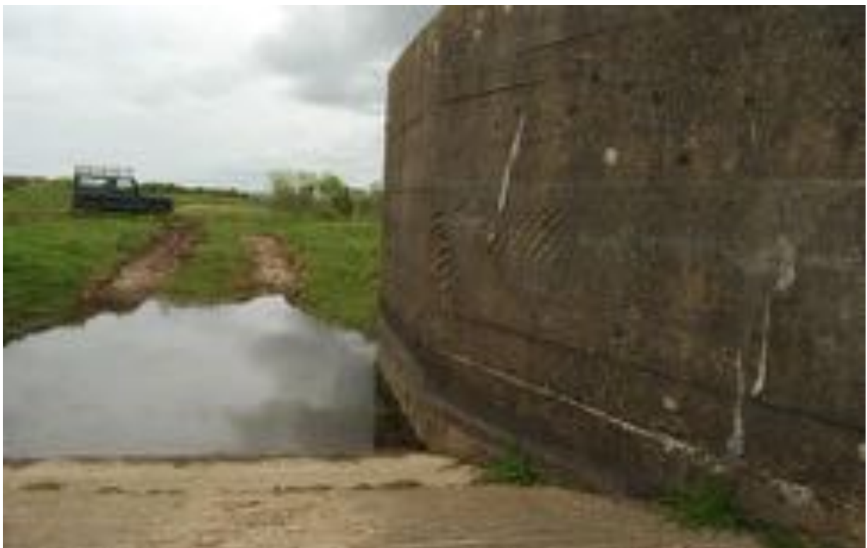
Concrete landing craft with tank rash — Braunton Burrows, Devon.
